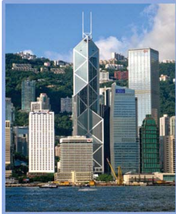
Figure 1 Bank of China Tower: Hong Kong
