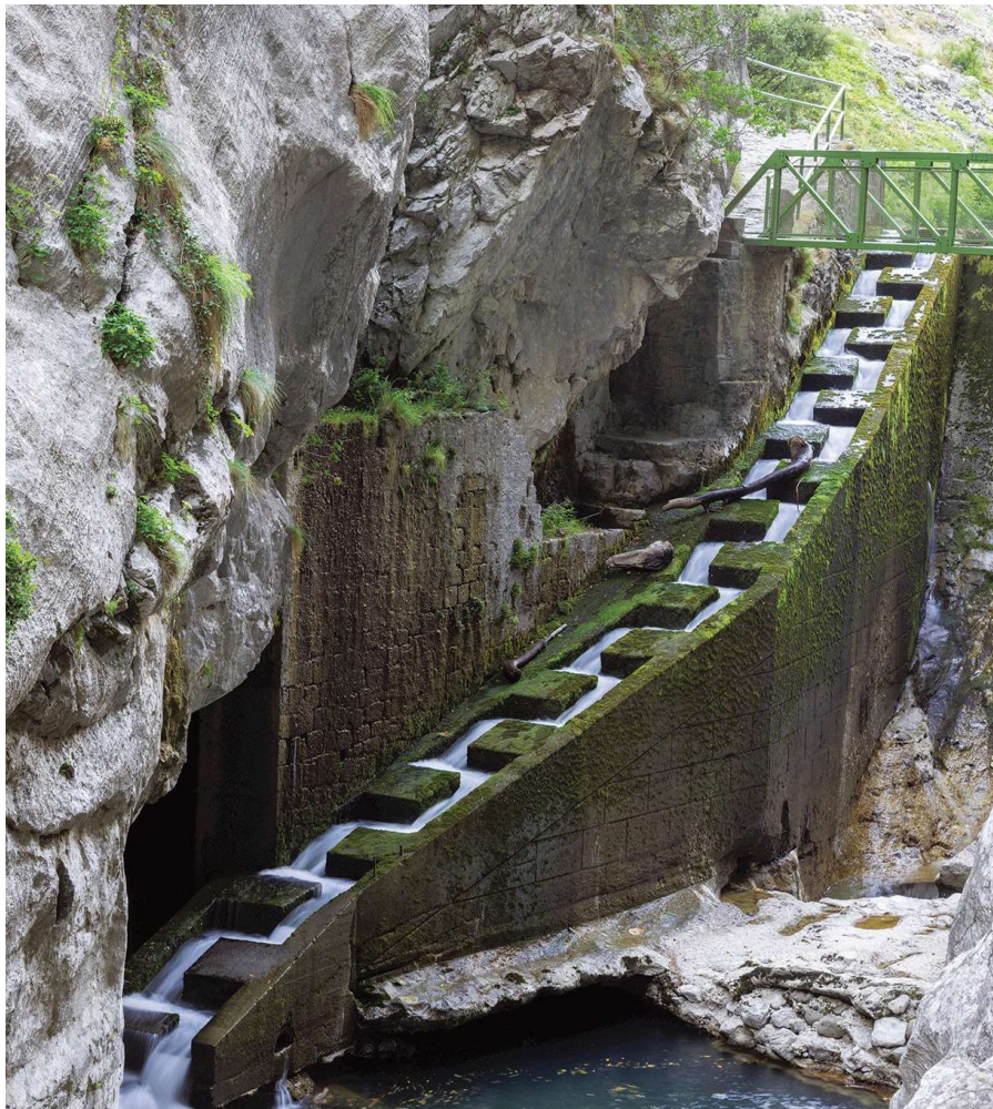
This is one example of a fish ladder. Fish swim up the ladder to get to the other side of the dam.
