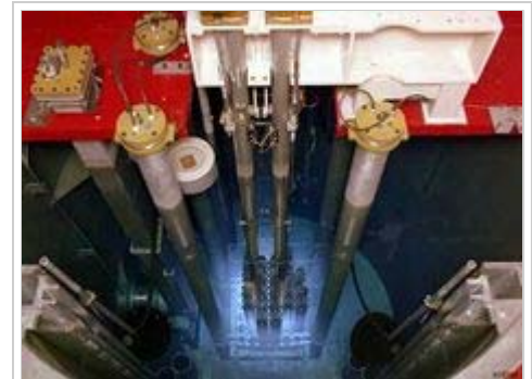
The blue glow in this "swimming pool" nuclear reactor is Cherenkov radiation, emitted as a result of electrons traveling faster than the speed of light in water.
