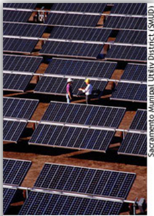
Photovoltaic technologies, like these flat-plate crystalline silicon arrays, can produce electricity even on cloudy days.
