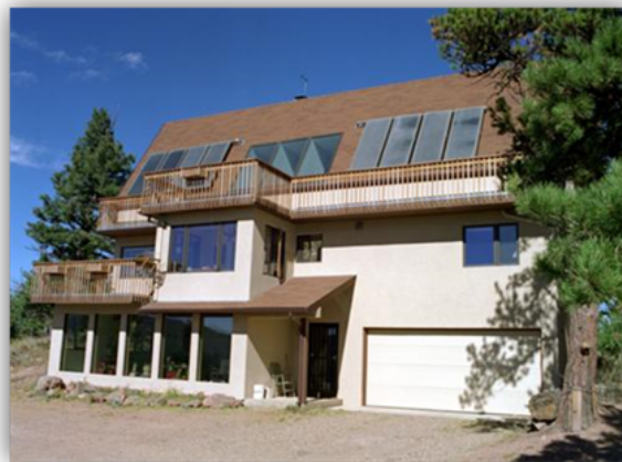
(above) This is an example of a passive solar home. Notice all the south-facing windows and the overhang above them
