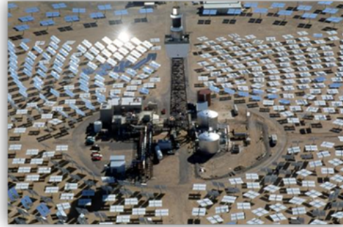
A solar power tower receives concentrated sunlight from the mirrors surrounding it. The heat warms the fluid inside the tower that is used to boil water to make electricity.
