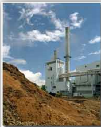
Biomass Power Plant - Photo credit: U.S. Department of Energy, Energy Efficiency & Renewable Energy Network (EREN)
