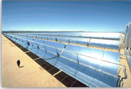
Solar parabolic troughs heat fluid in the tube in the center which is then used to heat water to produce steam to make electricity.
