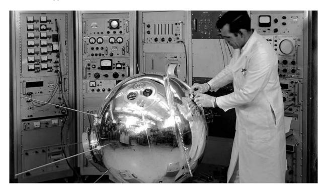
This is a photo of the Explorer XVII satellite. Weighing 405 pounds, this 35-inch pressurized stainless steel sphere measured the density, composition, pressure and temperature of Earth's atmosphere after its launch from Cape Canaveral, Florida, on April 3, 1963. Photo: NASA
